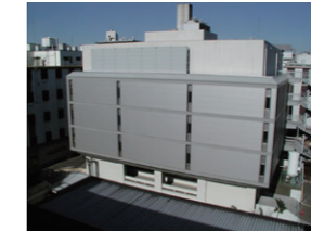
The building of the Laboratory Animal Research Center
